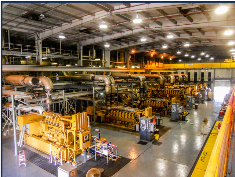
Inside the power plant. (6) 16-cylinder Caterpillar C280-16 generator sets @ 4.4 MW each (7000 hp @ 900 rpm) 350 gallons of diesel per hour per engine. Plus (1) 6-cylinder Caterpillar C280-6 – 1.8 MW (2700 hp @ 900 RPM)
