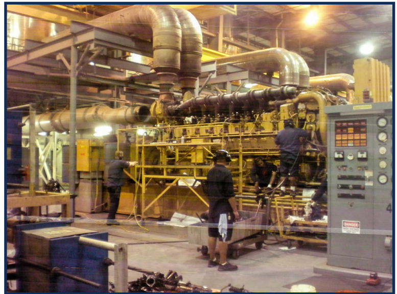
Inside the power plant. (6) 16-cylinder Caterpillar C280-16 generator sets @ 4.4 MW each (7000 hp @ 900 rpm) 350 gallons of diesel per hour per engine. Plus (1) 6-cylinder Caterpillar C280-6 – 1.8 MW (2700 hp @ 900 RPM)
